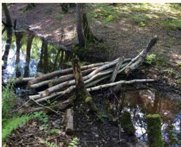
Ditch top flow diverters.
