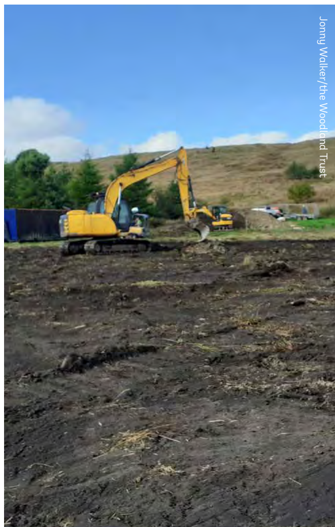
Creation of offline temporary storage area in progress.
